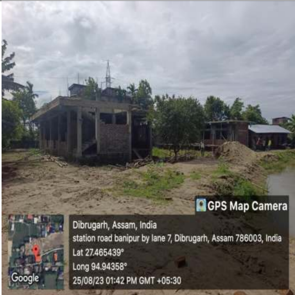
Progress of Boys' Hostel Construction Work at Banipur Campus
