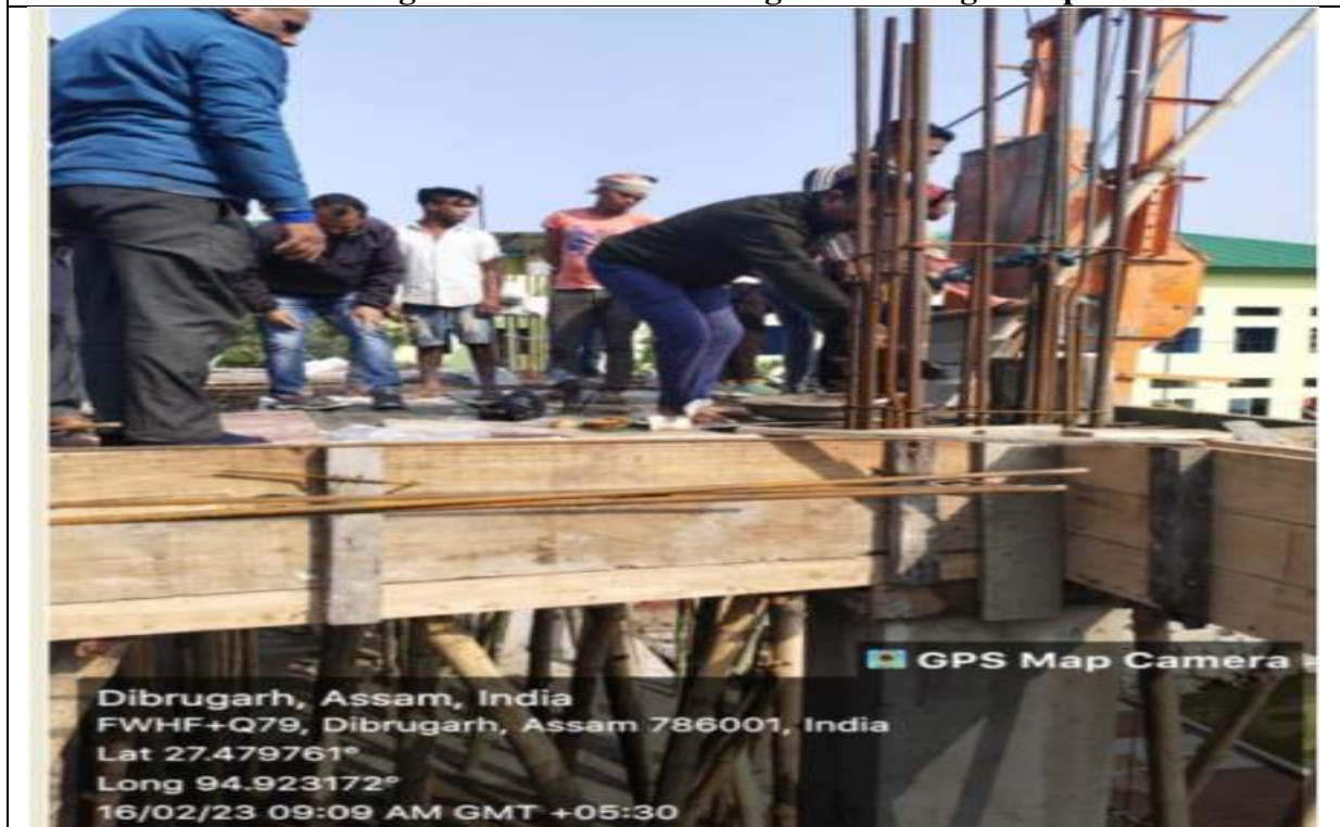
Slab casting of multi-stories building in the College campus
