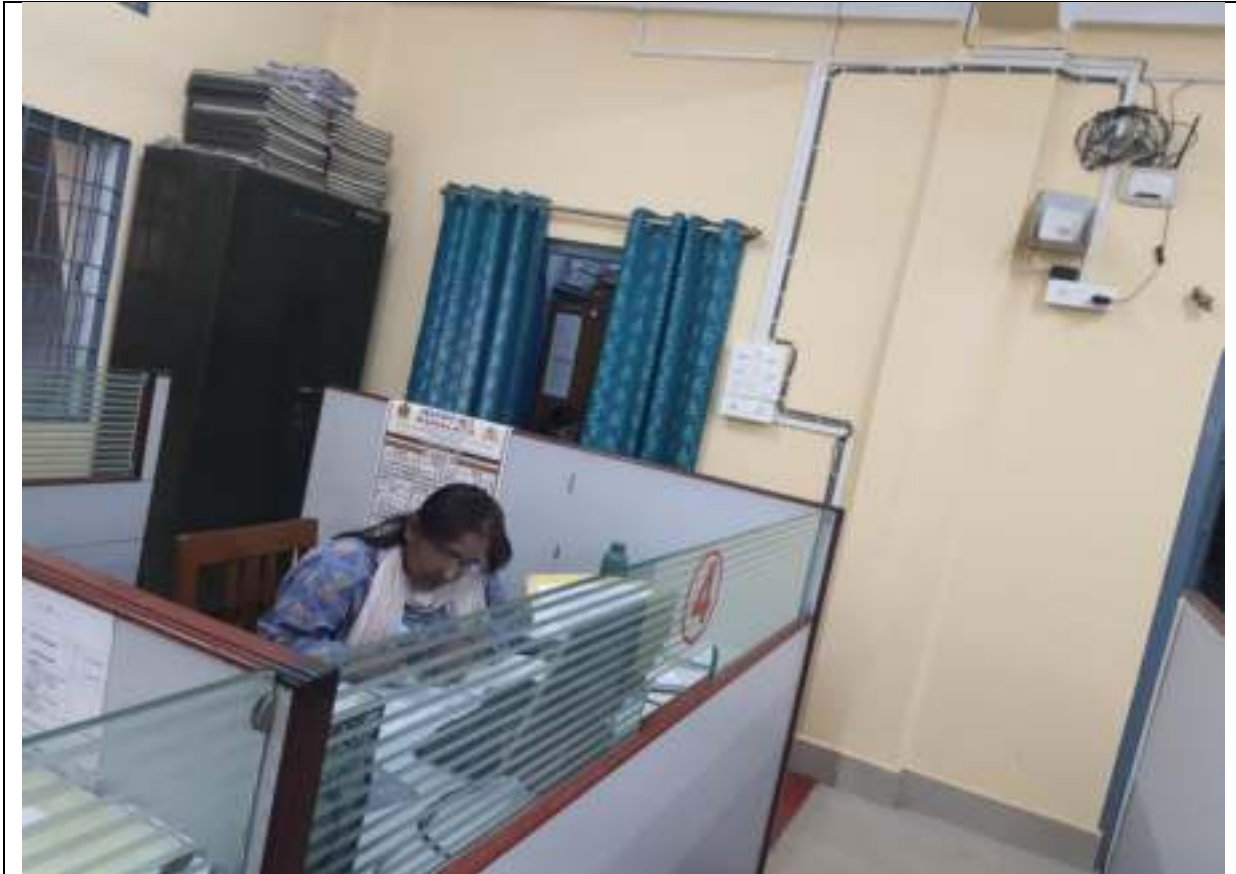
Modem and Router
