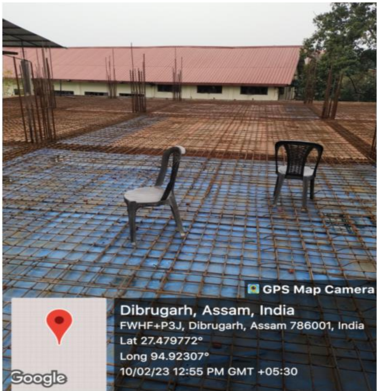
Construction work on new building
