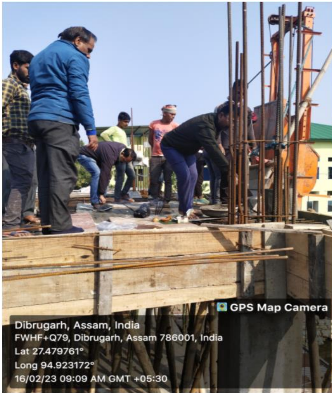
Construction work on new building
