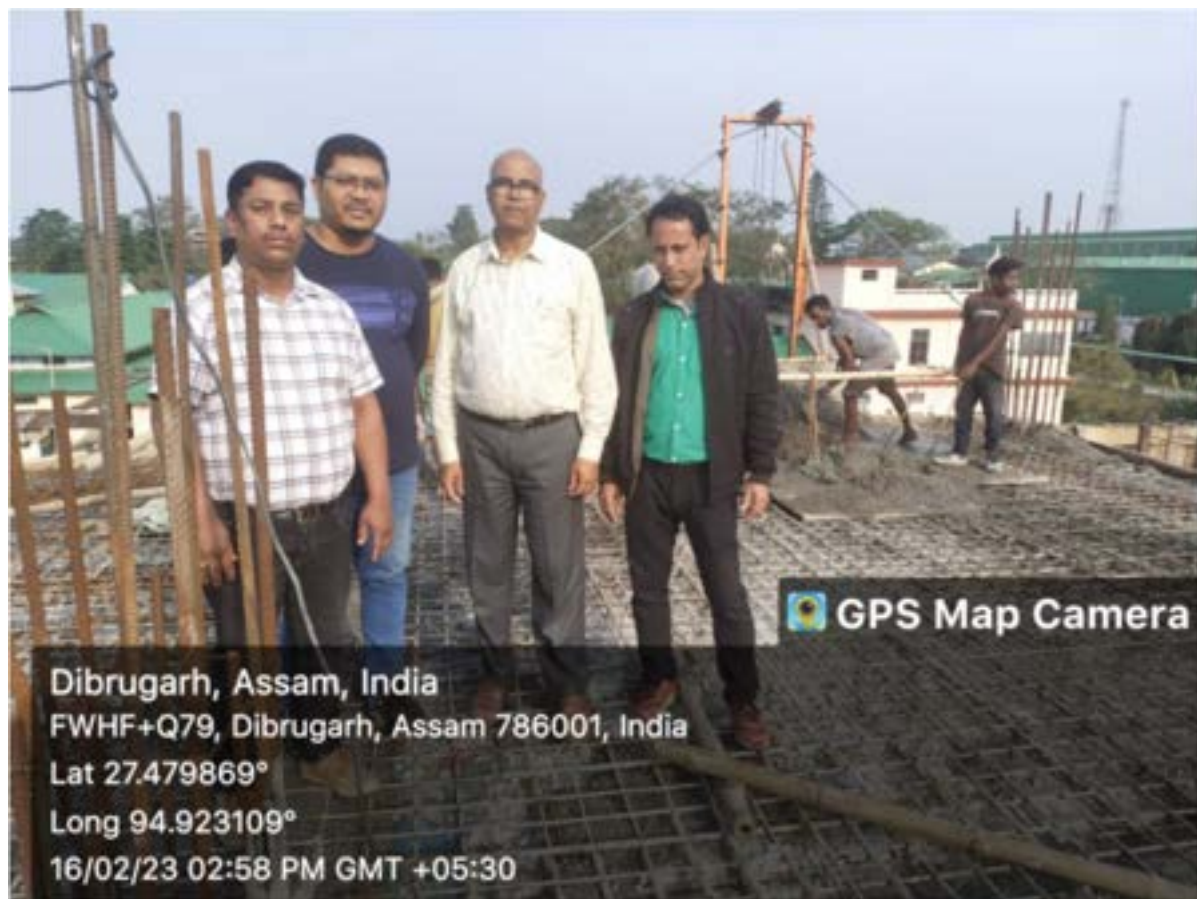
Construction work on new building
